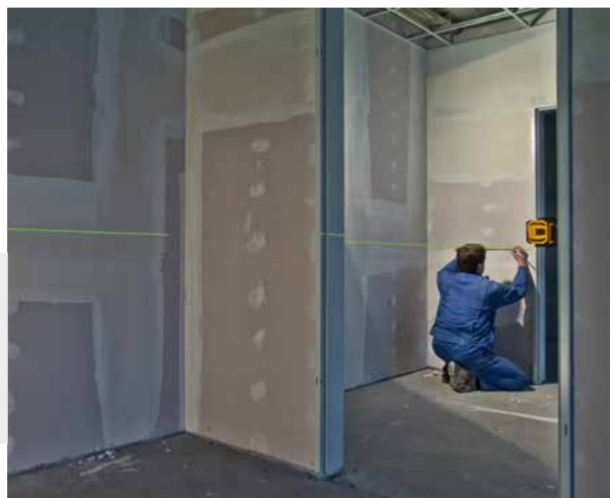
Optimum visibility – razor-sharp laser lines over the entire working area. The vertical laser line almost covers the entire room.
